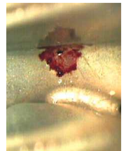
Figure 8.30 (b) Pitting corrosion in stainless steel 316.
