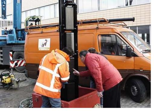
Inspection of a GeoThermic system by Westerlo, in the Netherlands. SWEP B45 BPHEs being lowered into the drilled well.
