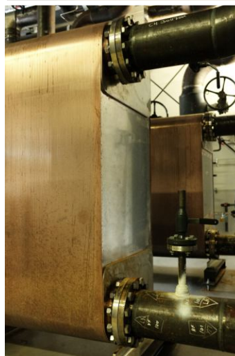
Two of SWEP's B649 installed in parallel. Each with 364 channel plates. Design pressure 25 bar at 120 °C and DN150 connections.
