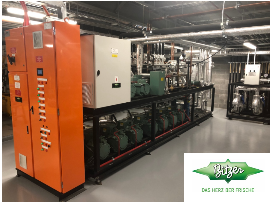
SWEP B12, B200T and B18 were used in this project. Chilled water production (+8/+12) via CO 2 thermosyphon. Suction superheat control for Low Temp compressors via liquid. Condensate subcooling via flash gas. Vapour condensing via R134a mechanical resilience unit. Heat reclaim to water via discharge gas for store heating.
