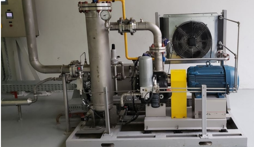
Biogas system where the SWEP B10T All-Stainless brazed plate heat exchangers are installed.
