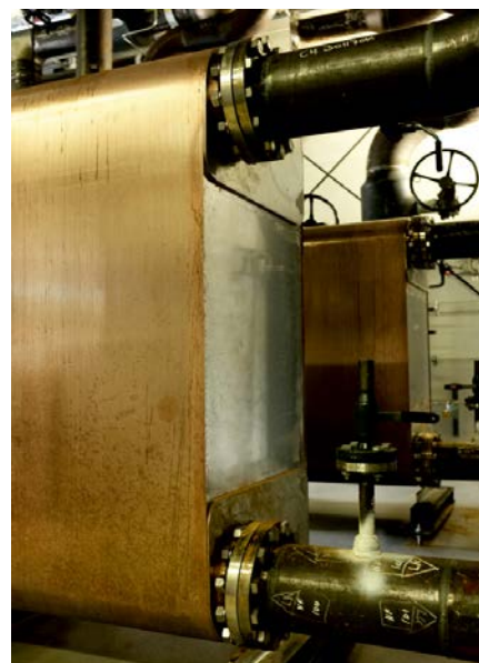
Two of SWEP's B649 installed in parallel.
