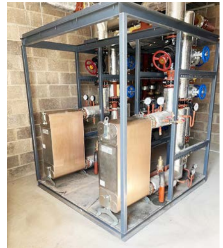
The future-proof substation solution, which uses SWEP B439Hx240 brazed plate heat exchangers.
