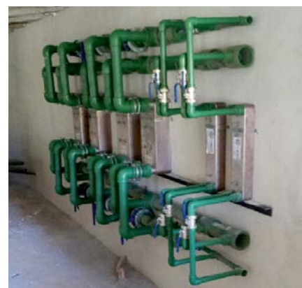
SWEP BPHEs, installed onsite, provide necessary heating.
