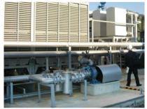
produced by the incineration process. The ORC system is used to remove the heat from the flue gas and convert it into electric power, which can be used onsite or sold locally.
